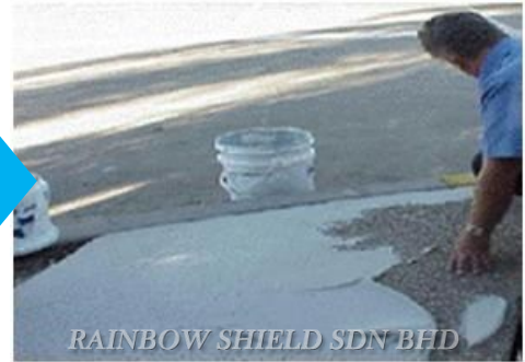
Apply base coat
