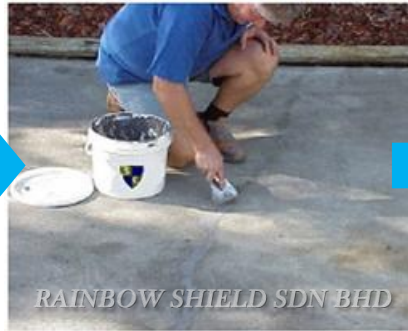
Apply Primer Plus and repair concrete cracks
